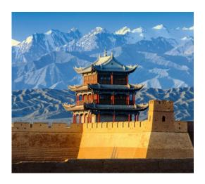
This military fort was constructed on top of the Great Wall. The wall itself was built using stone and clay bricks, but the fort was built out of stone and wood.
