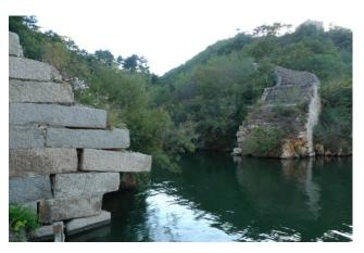
This section of the wall was built alongside a lake. The wall would have been taller than the lake when it was originally constructed, but since then the lake has flooded and caused damage to this part of the wall. Most of this section will need to be rebuilt in the restoration process, with an additional taller wall being built to prevent future flooding.
