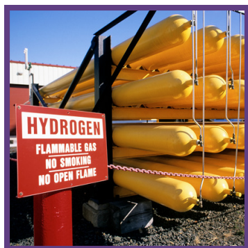
Engineers then built pipes and tanks to capture the hydrogen gas.
